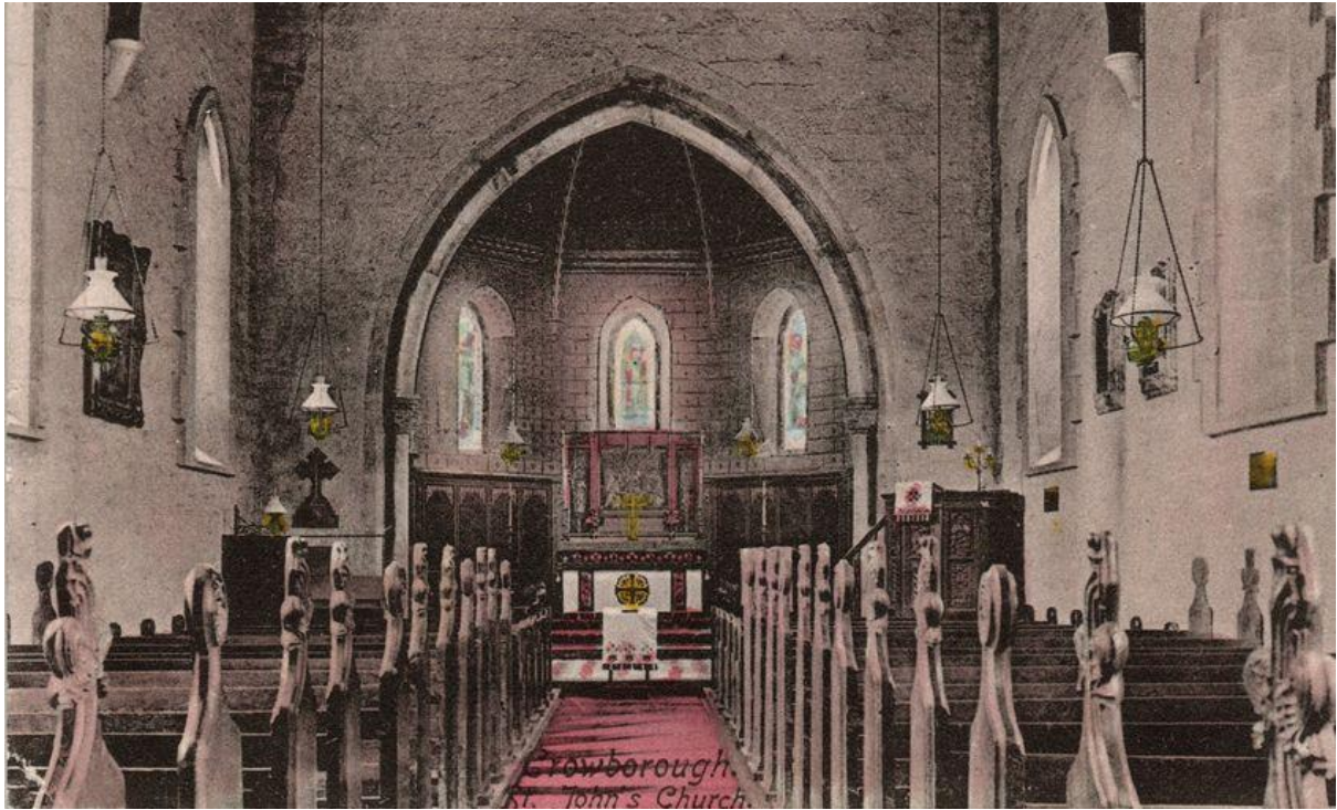
St John's postcard posted 1905 the stencilling on the chancel wall is just visible, together with the chancel panelling and carved pews. There is also evidence of significant damp on the walls.
